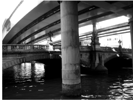
Photo-5 Nihonbashi covered by the Elevated Expressway
