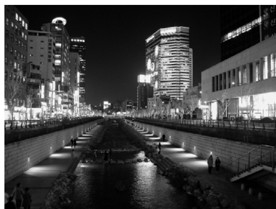
Photo-3 Restored Cheong Gye Cheon at night
