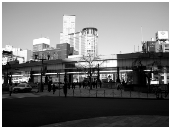
Photo-4 Nihonbashi covered by the Elevated Expressway
